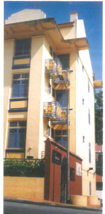
Cleverly concealed air-conditioning condensers behind timber grilles
