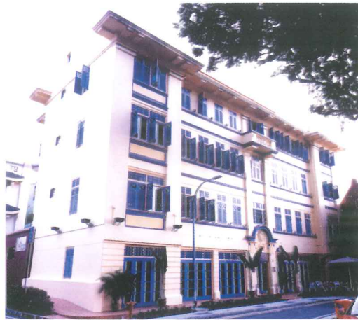
Restored front facade of the 4-storey Art Deco building
