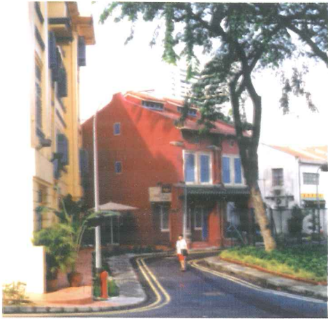
Original features of the 2-storey Early Style shophouses retained and restored
