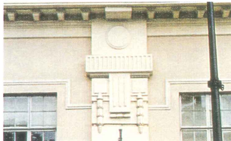
Rusticated column with moulded capital
