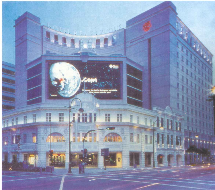
Well-balanced integration of old and new buildings
