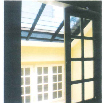
New airwell introduced to enhance the interior of a conserved terrace house
