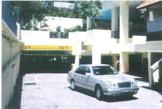
A new basement car park to meet the needs of the residents
