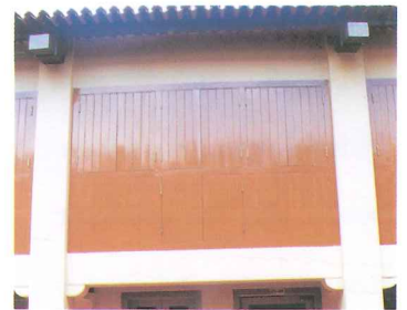
Rail and stile windows kept for reconstructed 2-storey shophouses at the rear
