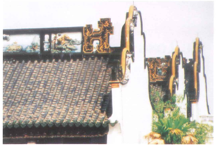
Main roof with concrete ridge frieze, gable walls and ornamental copings
