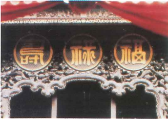
Decorative timber screen
