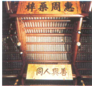
Timber purlins restored
