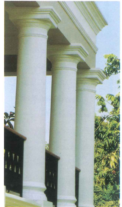
Circular columns with moulded capitals and bases
