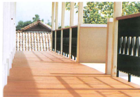
Balcony railing of original design
