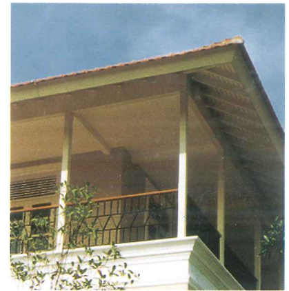
The restored overhanging roof further shades the balcony
