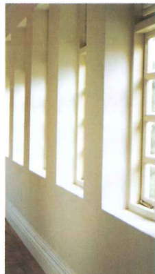
Casement windows viewed from the interior
