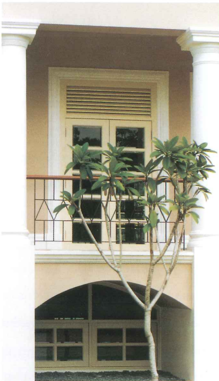
All external features including the basement arches were reinstated to original design
