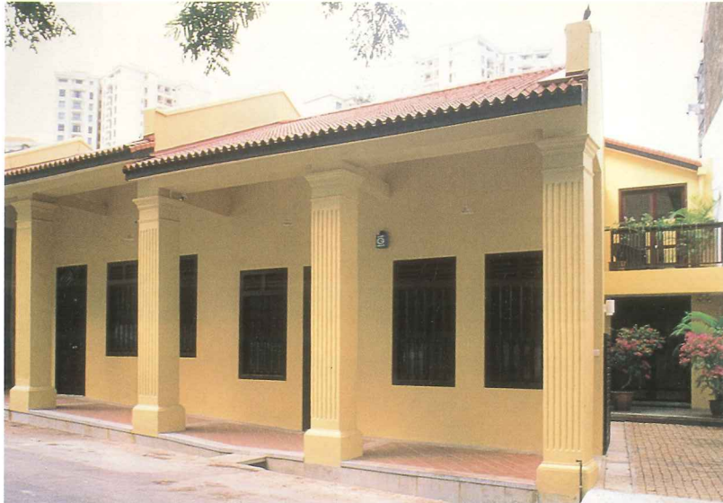
Single-storey warehouses restored into a traditional Chinese courtyard house
