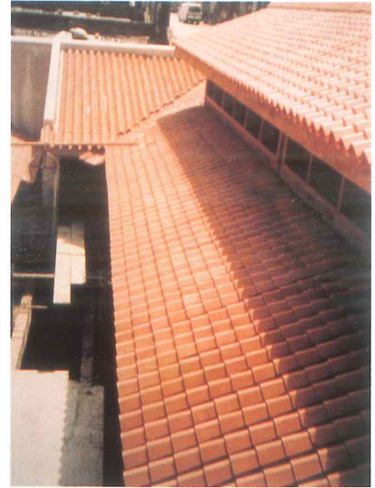
Jackroof to bring in light and air to building interior
