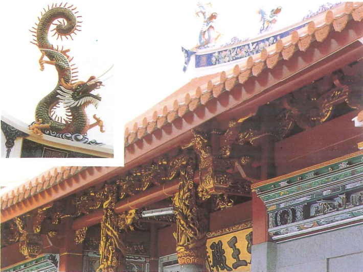
Restored ceramic ornament at roof ridge
