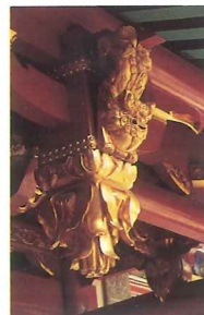
Decorative timber element
