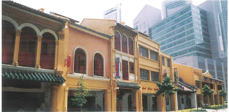
Restored conservation buildings of various architectural styles
