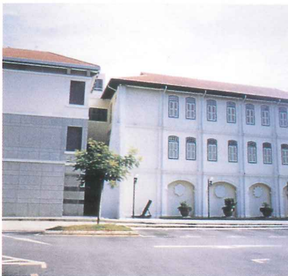
Horizontal cornice lines in old building pulled across to new extension
