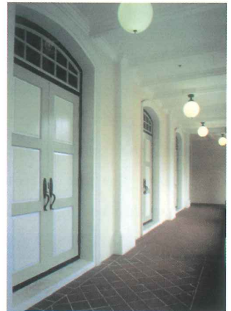
Restored timber doors at balcony
