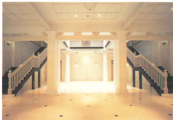
Atrium and staircases at main lobby restored to original design
