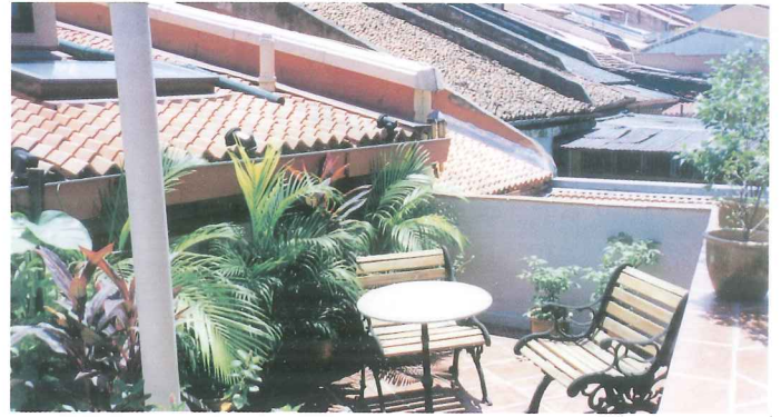
Roof terrace at rear roof mezzanine
