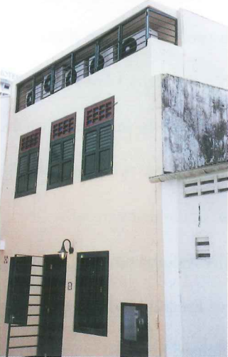
Air-conditioning condenser units neatly housed at rear extension
