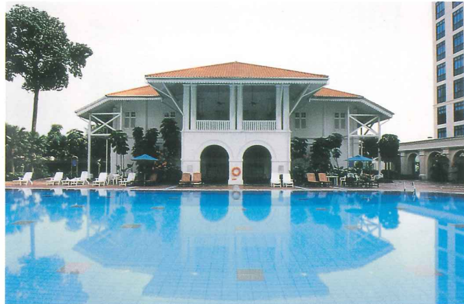
Restored club house overlooking the swimming pool
