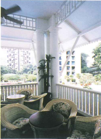
Open verandah with timber elements retained
