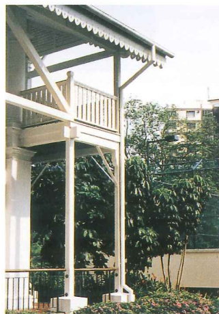
Eaves supported by timber post raised from the ground
