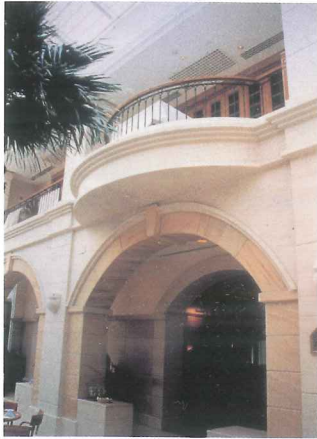
Details of arches
