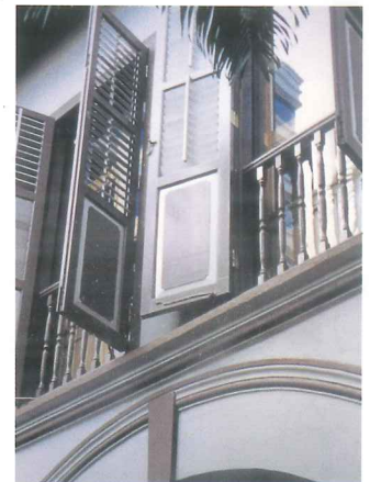
Timber windows restored and retained
