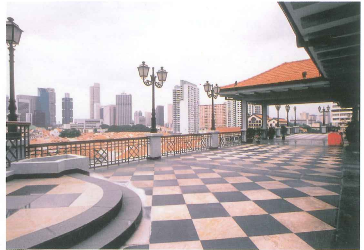
Sixth storey roof terrace
