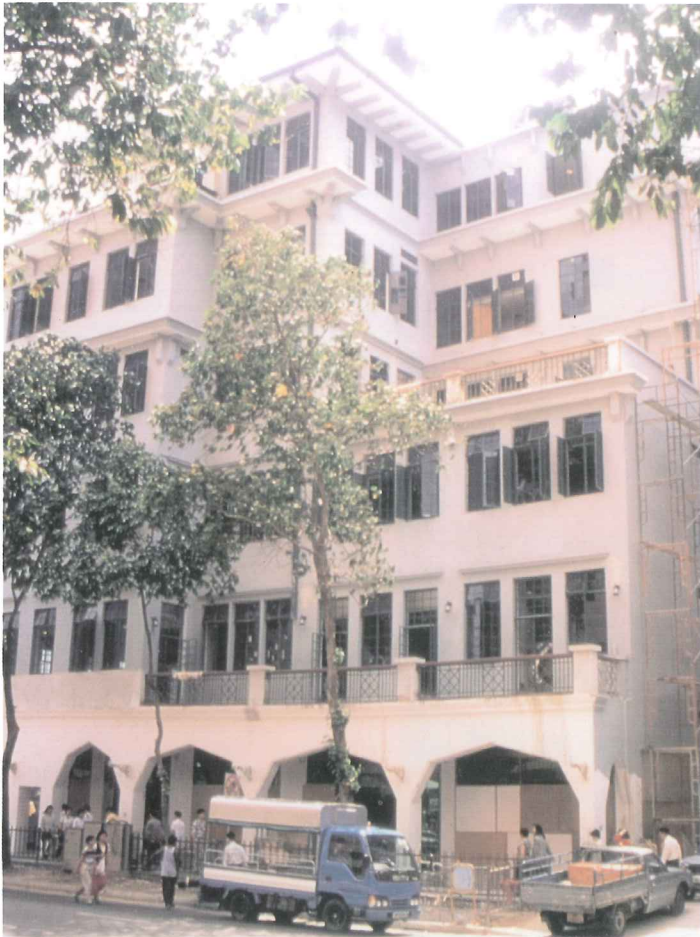
Side elevation showing the part six and part three Art Deco building
