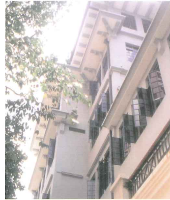
Original architectural elements restored
