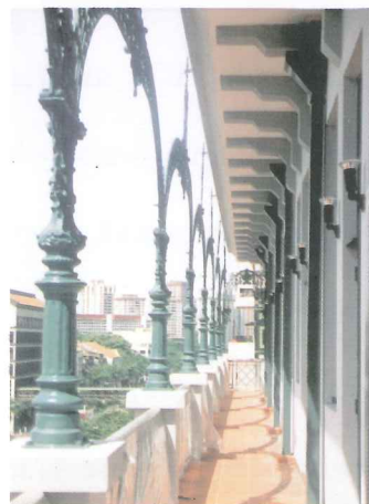
Cast-iron arches retained and carefully restored
