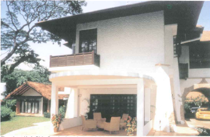
The patio outside the Dining Room is reinstated to its original design (by Swan & Maclaren 1951). Towards the left is a glimpse of the Rain Tree which was conserved and the new extension curve-block
