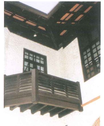
Original balcony restored
