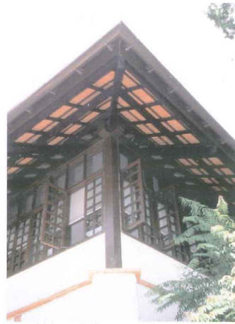
Exposed timber roof rafters
