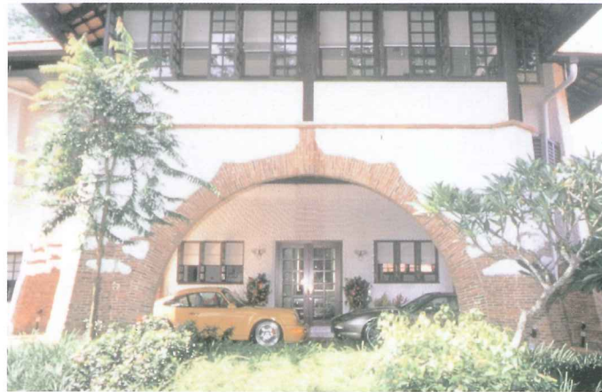
Brick arches with keystone & fair faced brick base
