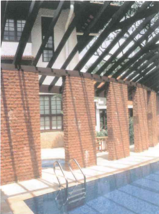
The Main House looked through the exposed timber rafters of the extension curve-block. The new extension is built with load-bearing rock-face bricks sympathetic to the Main House
