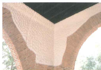
Rough cast plaster
