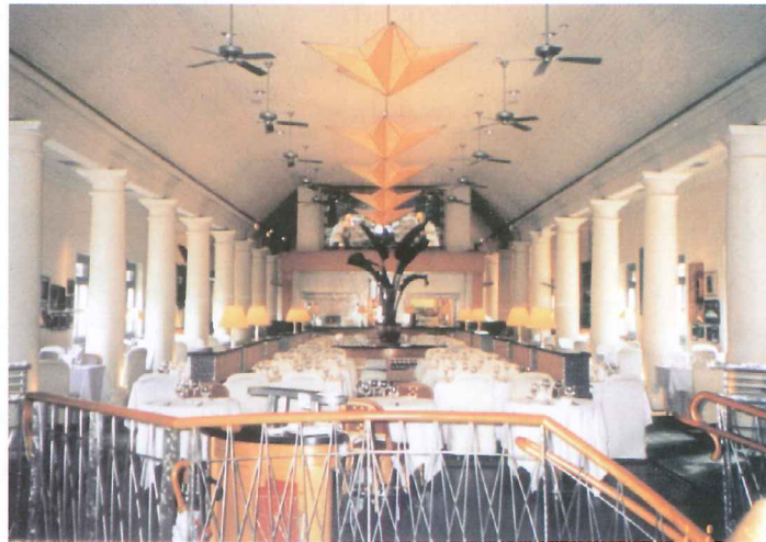
Interior columns & ceiling boards retained, restored, and replaced
