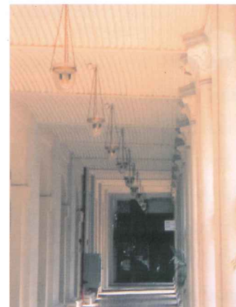
Restored corrugated ceilings immediately behind Caldwell House
