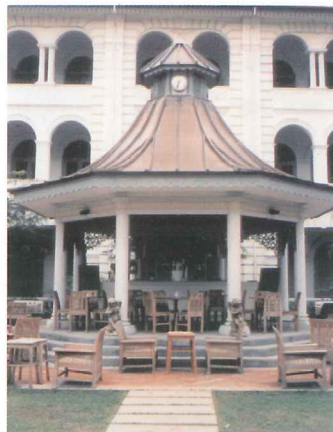
Pavilion added to enhance ambience of the place
