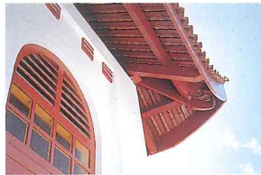
Restored up-turned roof eaves
