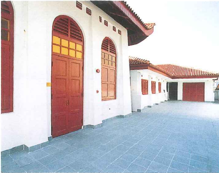
Restored original bell tower used as a prayer pavilion
