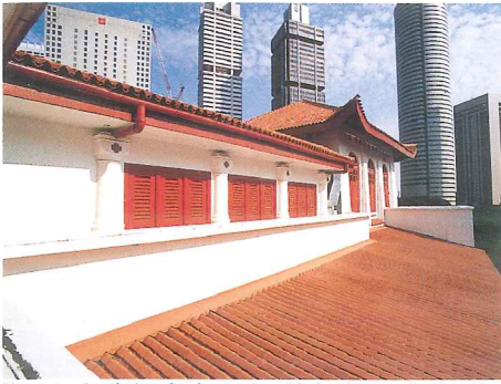
New extension designed to harmonise with the old by replication of architectural elements
