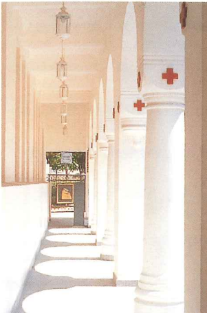
Retention of external verandah with its alternating circular and square columns to articulate the corridor space
