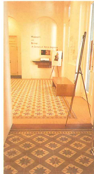
Old concrete tiles (foreground) carefully preserved
