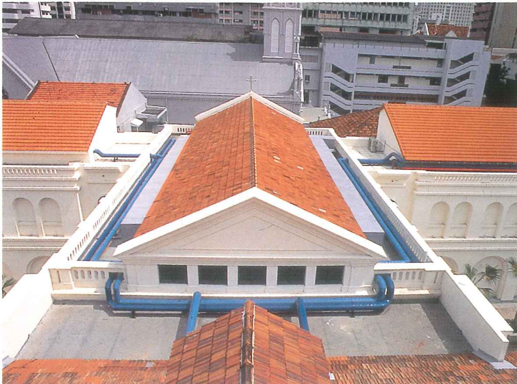
Service pipes and air-conditioning ducts properly concealed behind roof parapet walls
