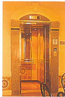
Modern intervention - elevator to serve the upper storey
