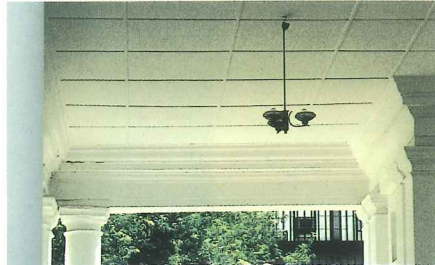
Simple ceiling grid pattern at entrance porch
