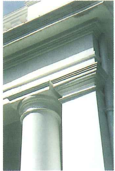
Circular columns with Doric capitals, shaft and base
