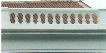
Parapet with turned-stone bottle balusters retained
