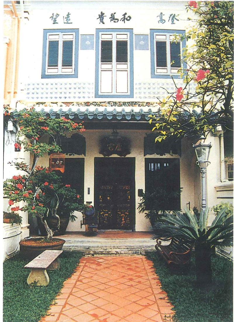
Main two-storey facade and forecourt restored to original details and finishes
