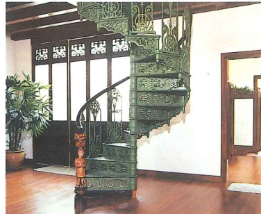
A new cast-iron spiral staircase introduced to harmonise with the older elements of the shophouse
