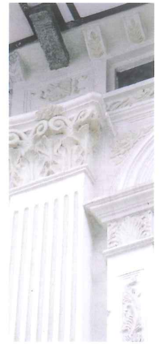
Fluted brickwork pilaster sensitively restored
