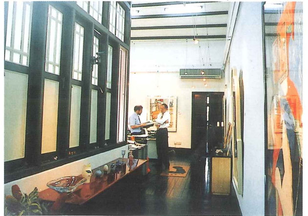
Passageway at second storey capitalises on the alternating naturally-lit space created by the airwell
