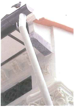
Interesting details at roof eaves
