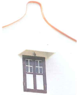
Coping at gable wall brings out the beauty of the shophouse
